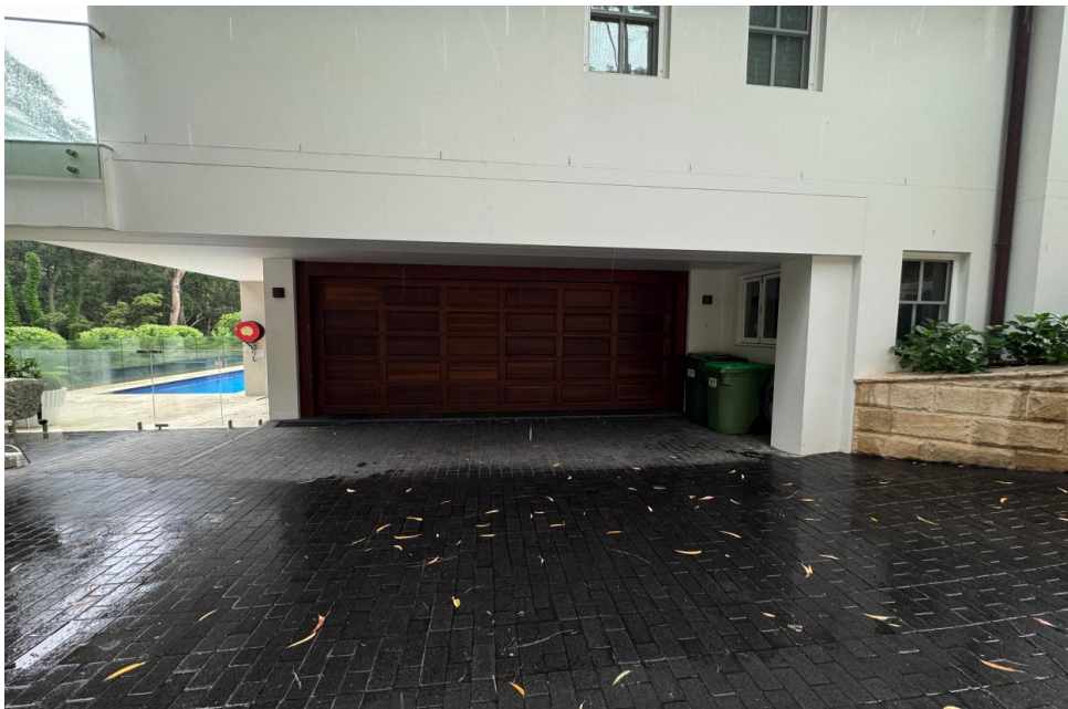
Figure 4: Existing garage looking east
