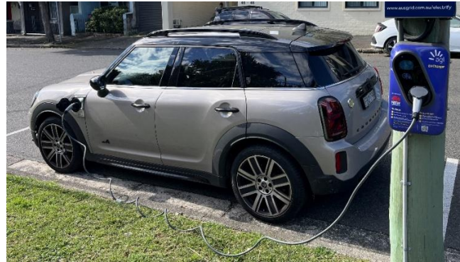
Figure 4 Example pole-charger in use within Inner West Council LGA
