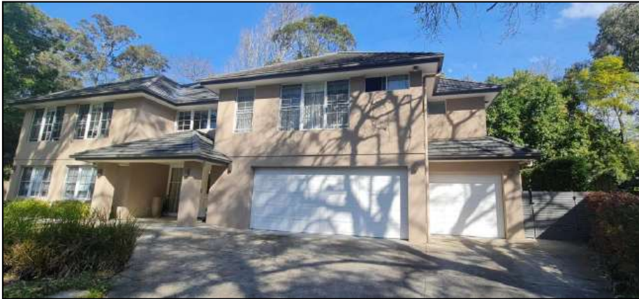
Figure 2: Existing building as viewed from Mahratta Avenue
