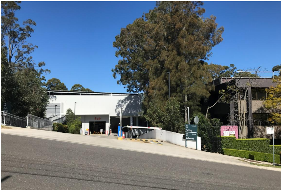
Figure 5: Bunnings trade entrance and secondary customer egress at left; subject site at right
