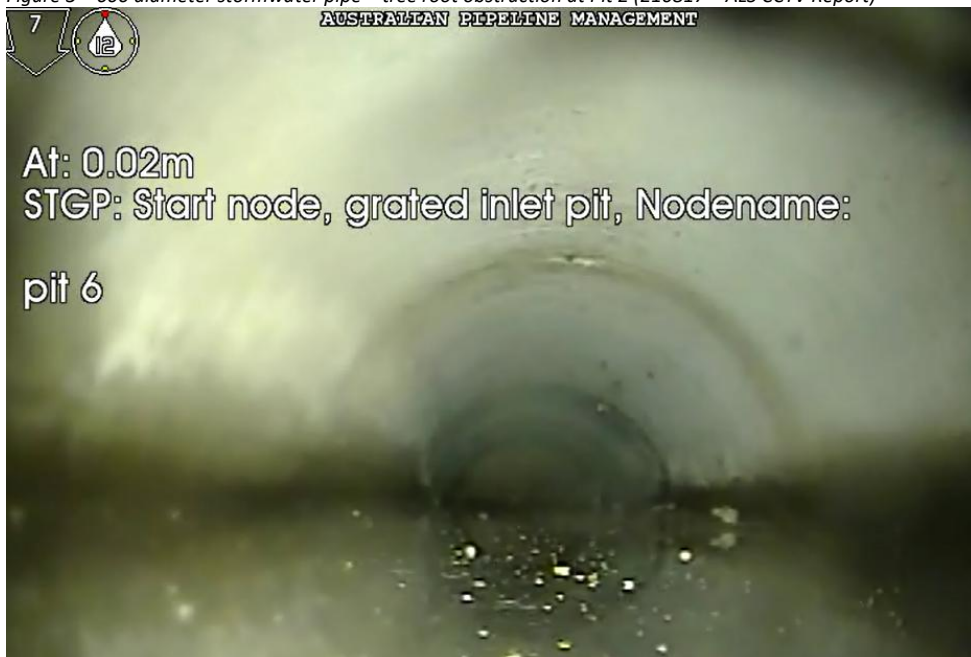
Figure 4 – 600 diameter stormwater pipe – Pit 6 looking to Pit 2 (210817 – ALS CCTV Report)
